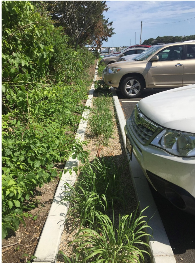
Figure 4b - Constructed Wetland: Stormwater flows into the wetland and then moves laterally through the root zone which is constantly saturated providing excellent treatment.
