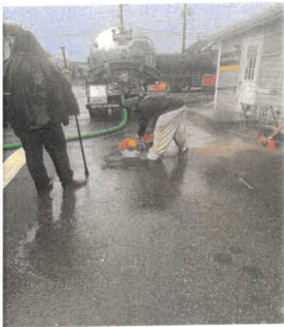
Cutting drive way to gain access to old solids tank/grease trap
