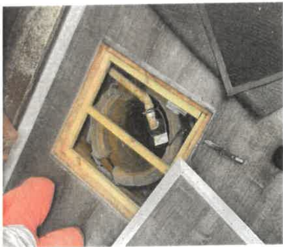
Sump pump located under a trap door in the floor covered with carpet.
