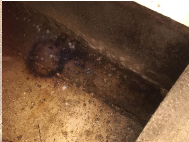
Circular mark is location of old pit and external weld
