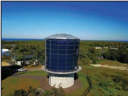
Our new tank is located on High Point Lane. Its capacity is 350,000 gallons. Its chief importance is fire protection redundancy.
